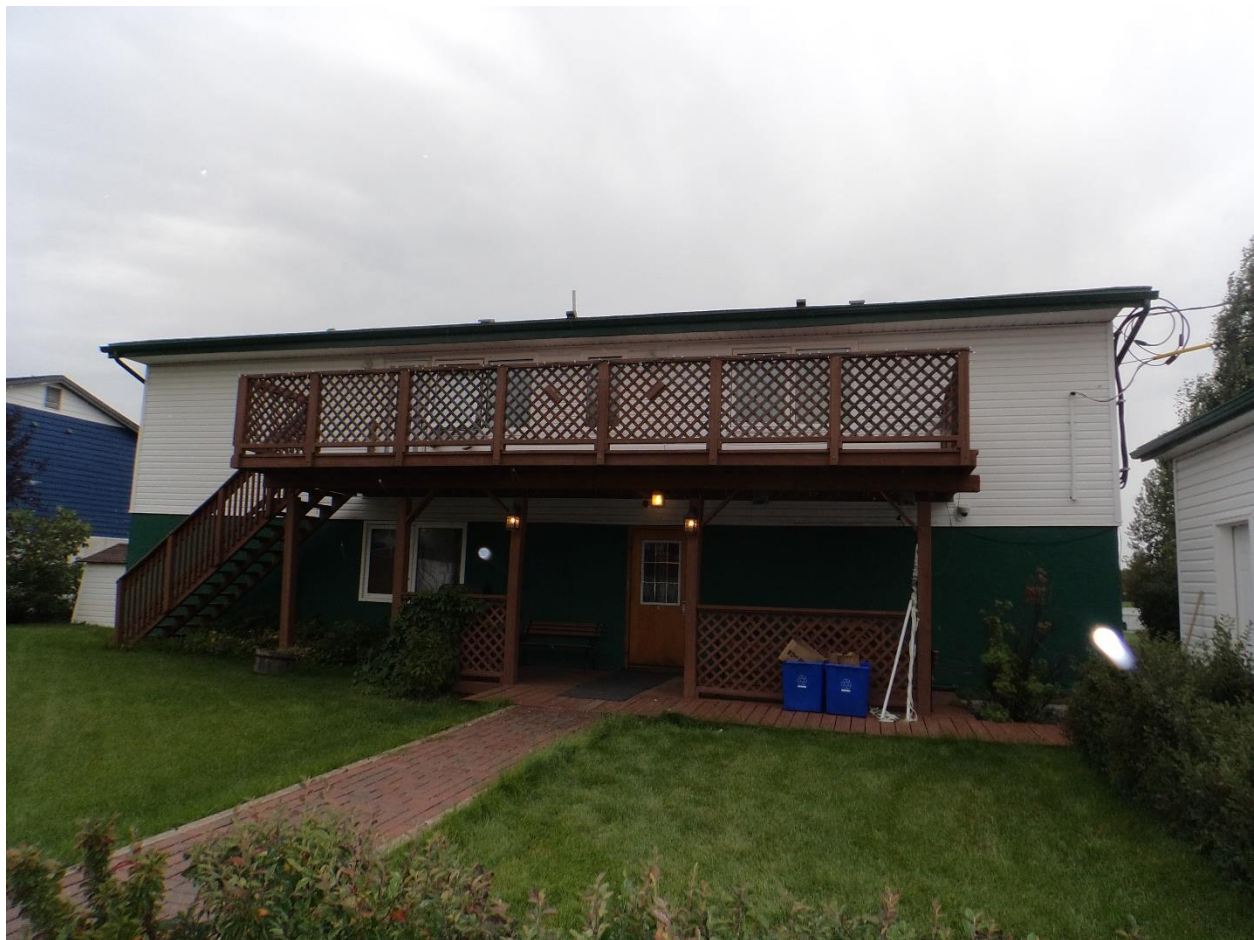
95 Cree Road House
