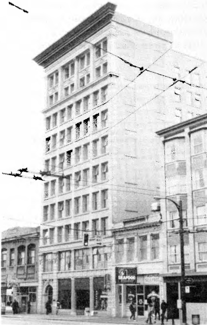
Tellier Tower at 16 East Hastings Street is across the street from DERA's offices. This "Class B" Heritage Building has received numerous architectural awards for the quality of the restoration.
