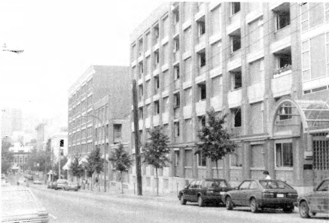
On the right is the south face of the Four Sisters Housing Co-operative. On the left is the 85 unit Columbia House project which is managed by the Affordable Housing Advisory Association. The Four Sisters courtyard and childrens' play are is between the two projects. The 153 unit Four Sisters Co-op consists of new construction and the rehabilitiaon of an existing building.
