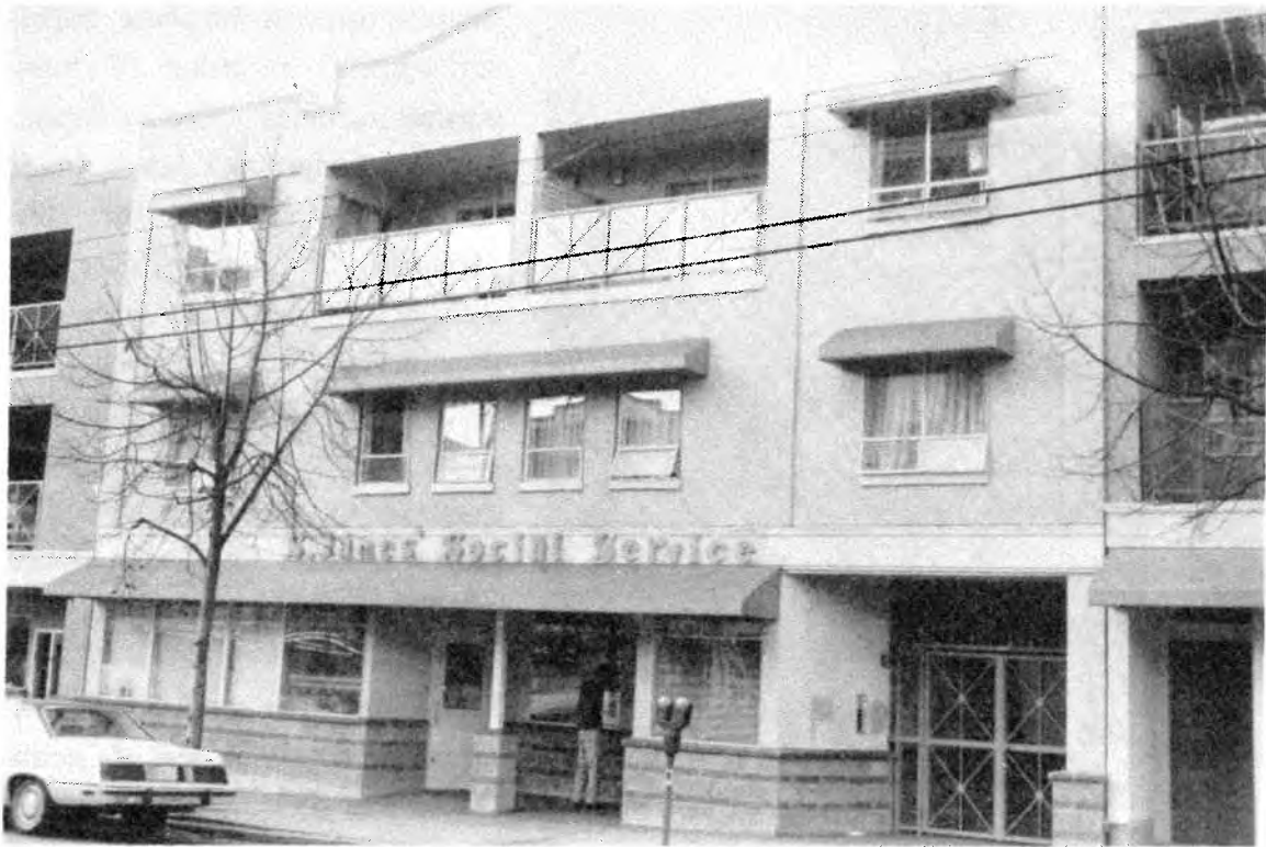
Cecilia House is built above the busy offices of St. James' Social Service Society.
