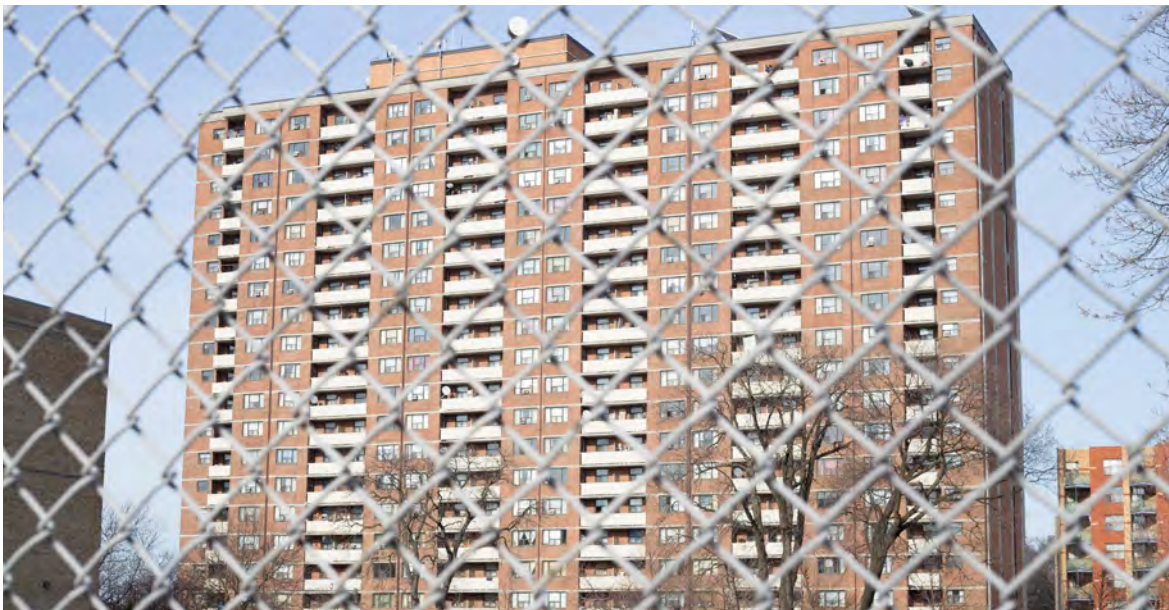
An apartment building Toronto, ON. (photo by Shane Fester)
